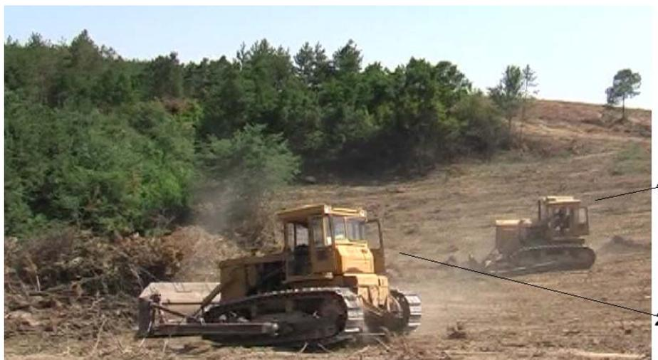
**Figure 1: Site preparation picture: 1 – Ripping aggregate – D-513A uprooter-ripper with T-170 crawler tractor; 2 – Bulldozer aggregate – DZ-27 dozer with crawler tractor T-170**
